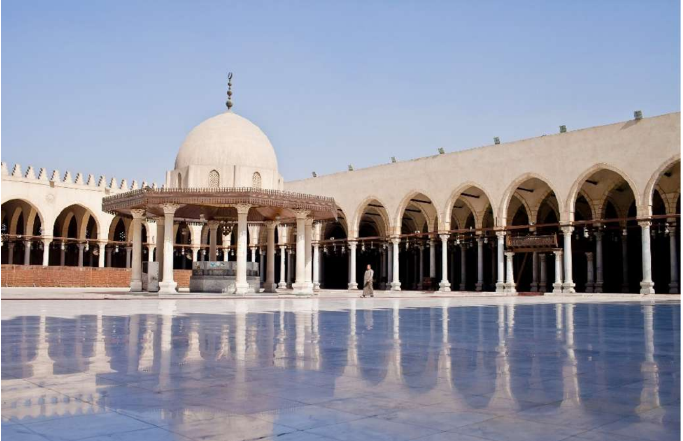
Figure 04: Mosque of Amr Ibn al-As in. Source: Ulama, n.d.
