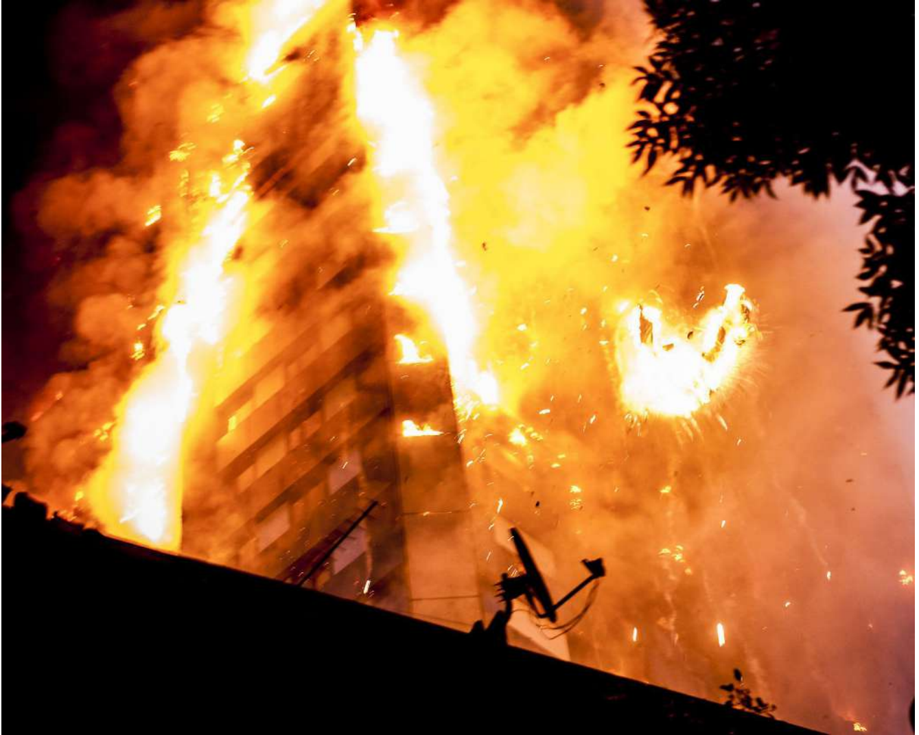
Figure 20: Fire accident in the Grenfell Tower. Source: Lawyer Monthly, 2017
