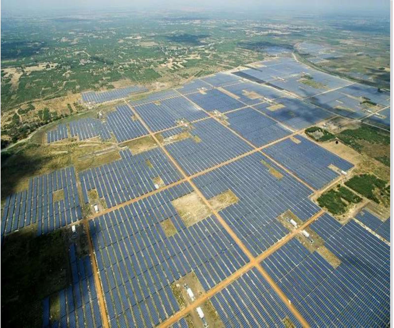
Figure 06: Solar panel installed in Karnataka. Source: Solartoday.co.in, 2016
