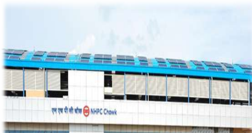
Figure 15: Solar on roof top. Source: Delhi Metro, n.d.
