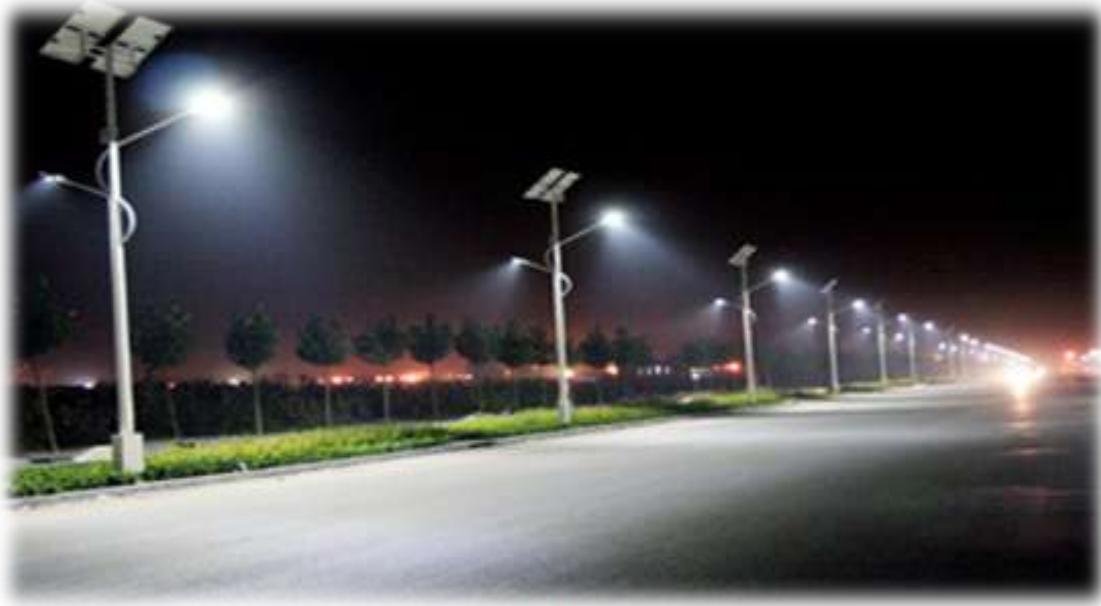
Figure 18: LED Solar Light system. Source: Solar Street Light, 2018
