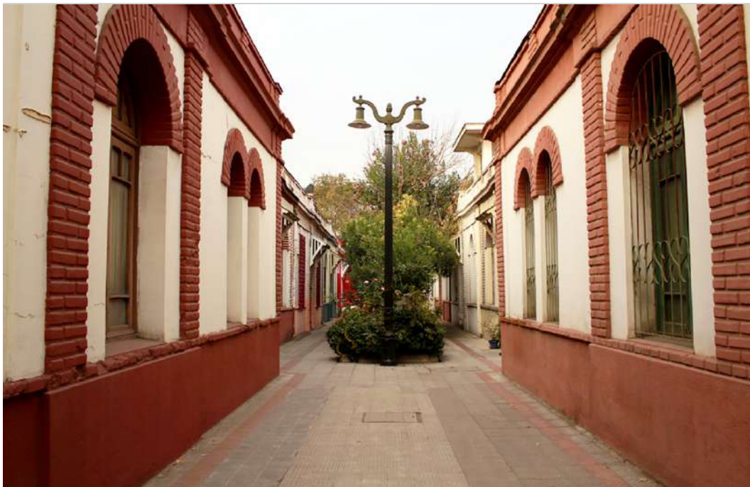
Figure 28: Continuous facade and the central open space in a two-storey cité for middle-class families. Source: Begining, University Bernardo O'Higgins
