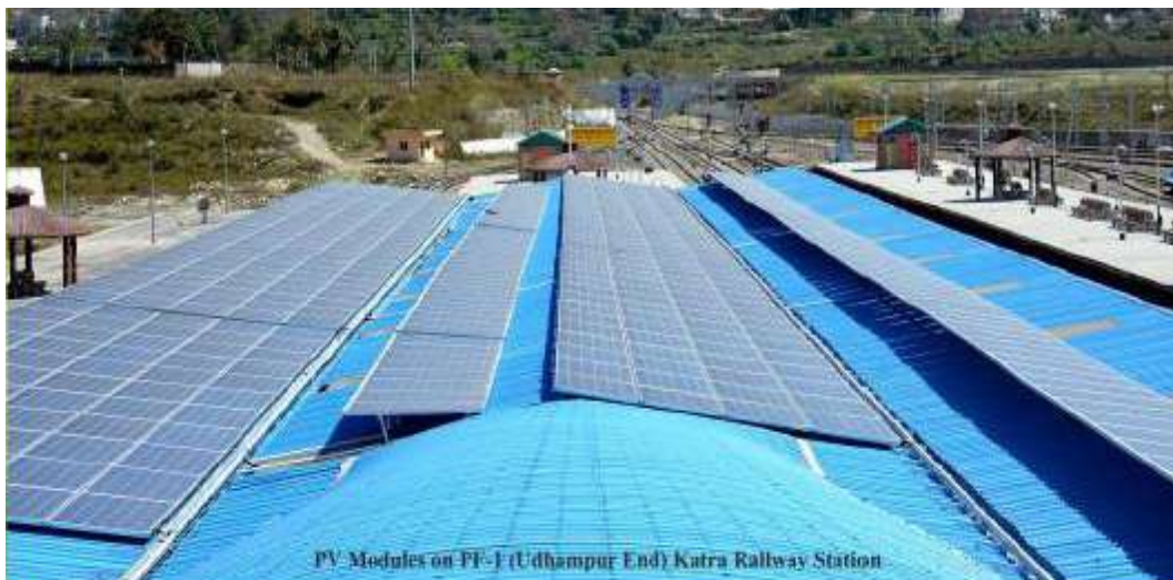
Figure 12: Solar Roof Top, Jammu, India. Source: Railway I. , 2016
