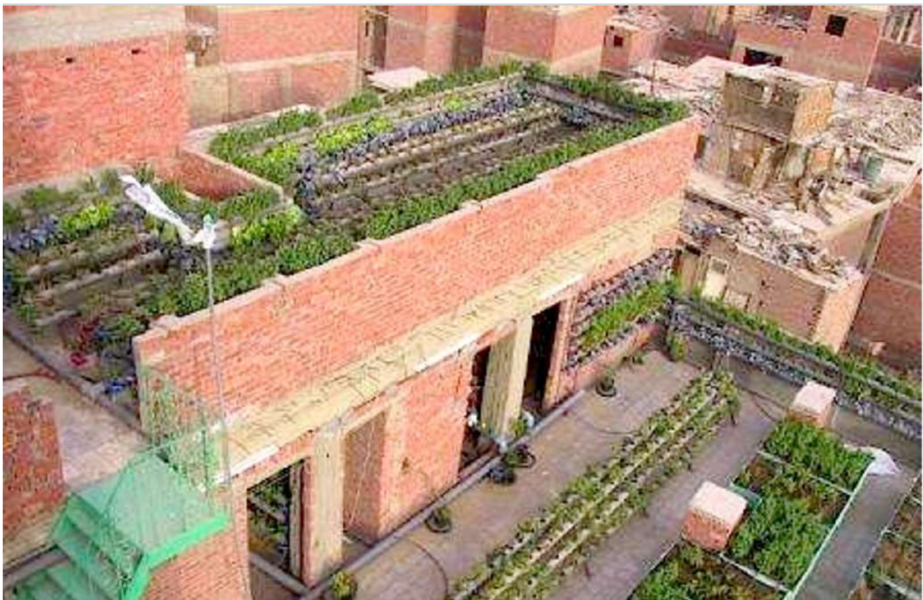
Figure 18: Roof Garden in Cairo. Source: Cityfarmer.info, 2018
