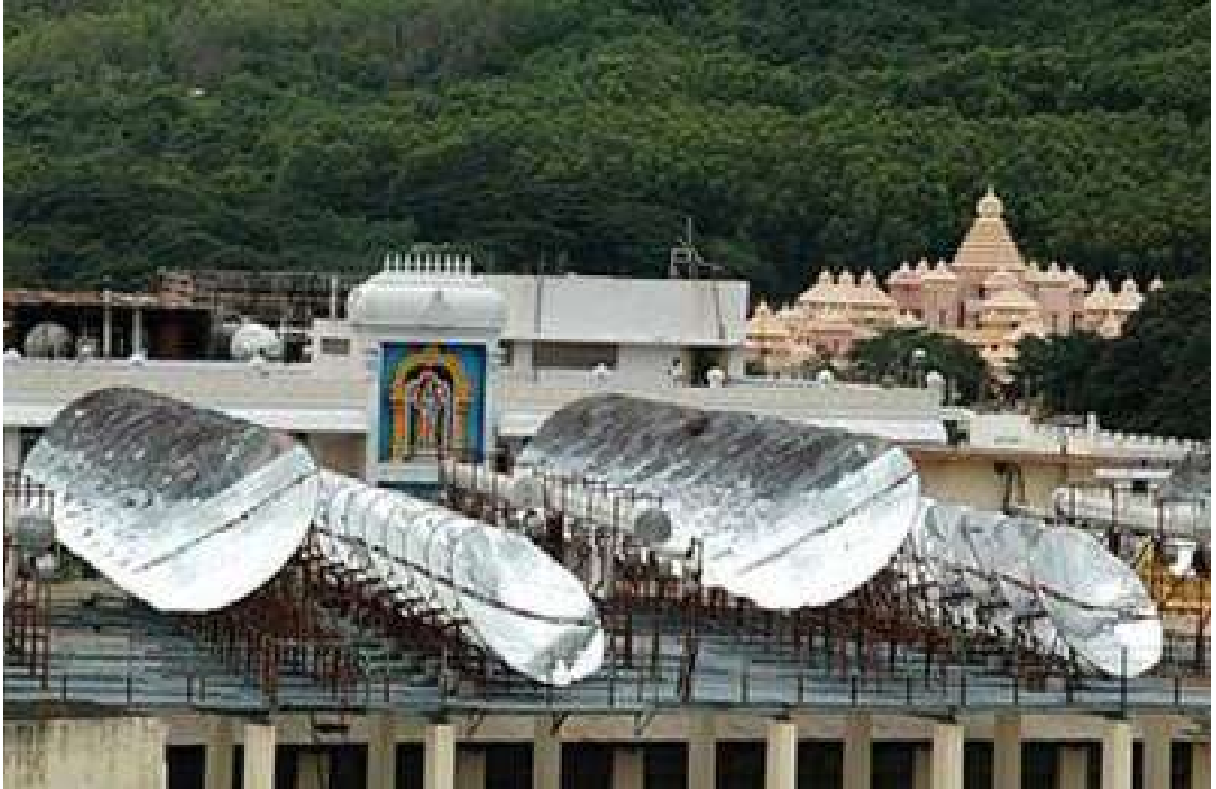
Figure 07: Solar panels installed at the Tirupathi Temple. Source: Terienviis, 2015
