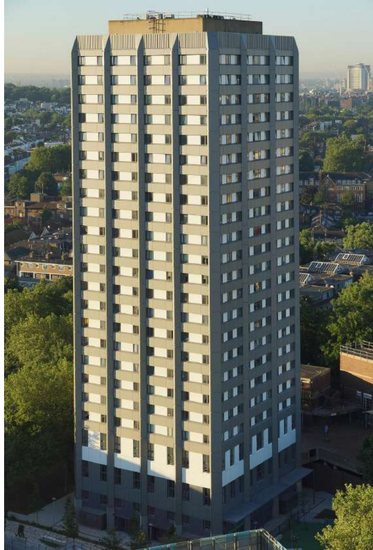
Figure 18: Grenfell Tower. Source: Grenfell Tower, North Kensington, 2015
