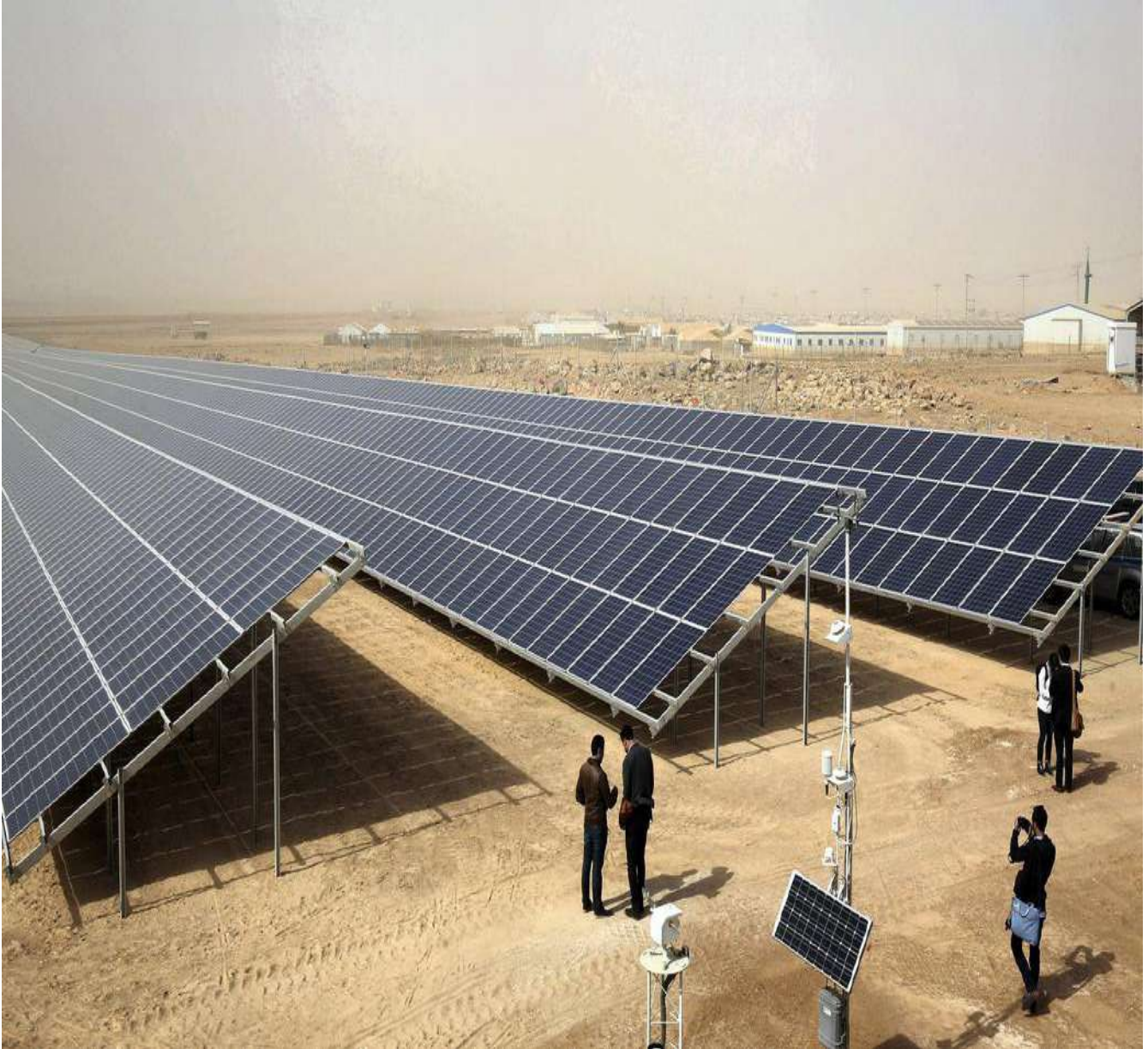
Figure 12: World's biggest solar power plant for a refugee camp opens in Zaatari. Source: Luck, 2017
